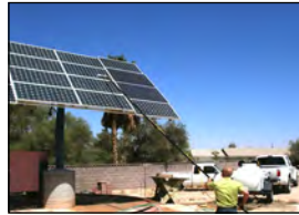
SOLAR PANEL CLEANING
